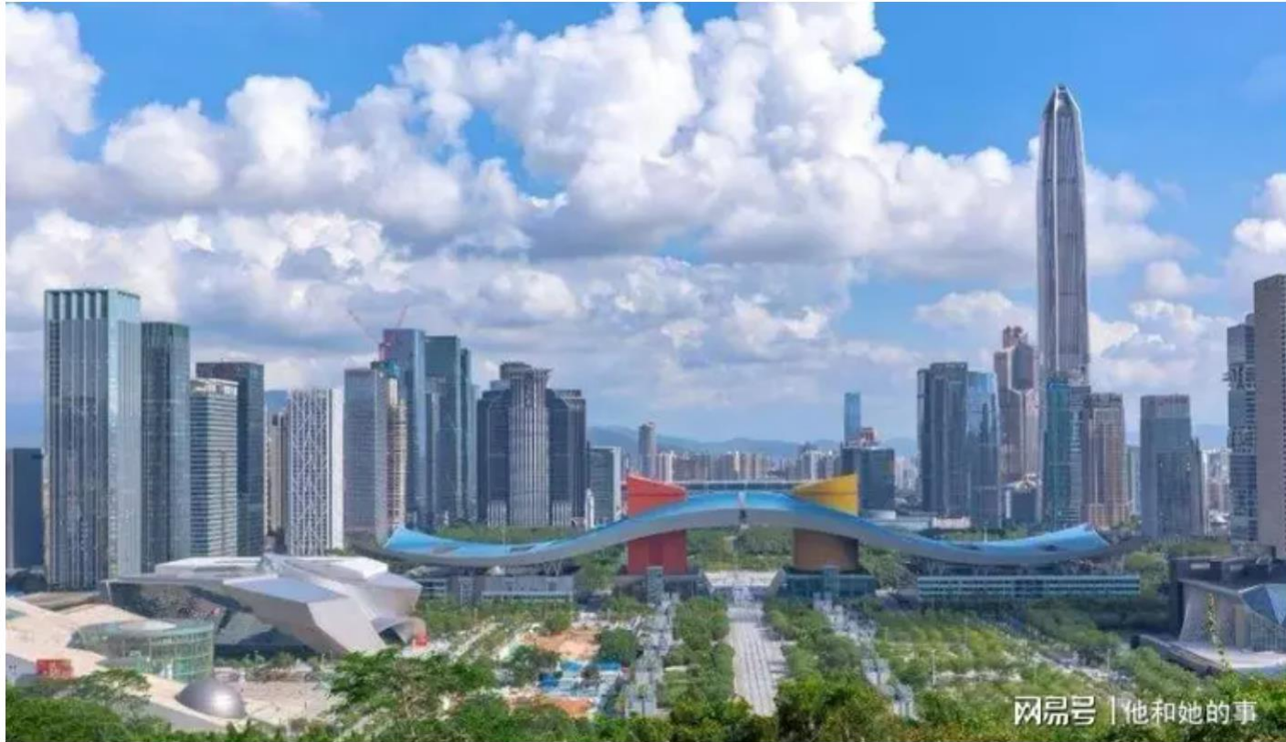
Meteorological Gradient Tower Shenzhen Ping An Building
